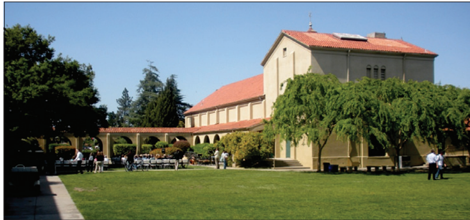
Figure 2-2: Theatre building on the school campus
