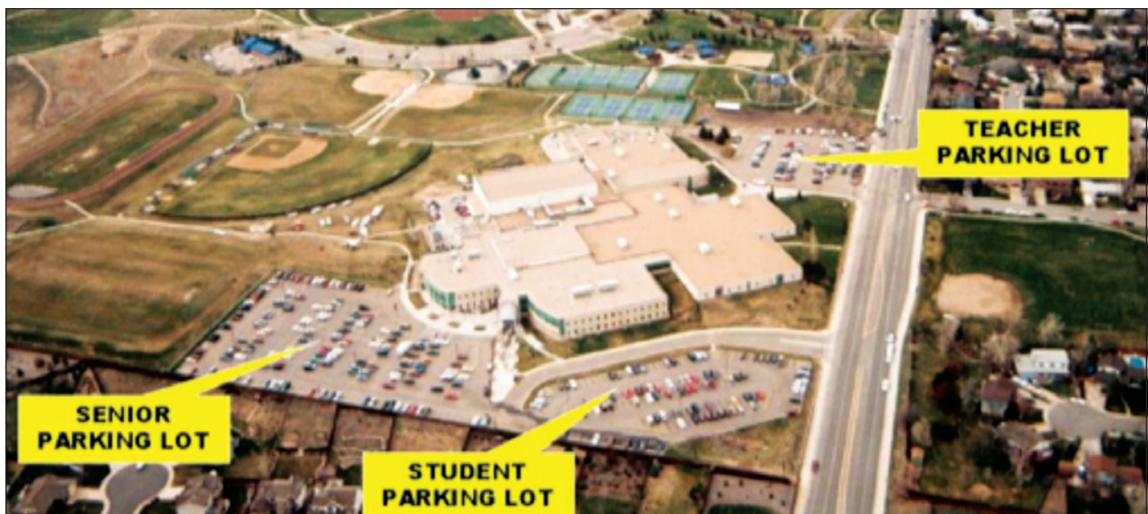
Figure 3-18: Aerial view of Columbine High School grounds
